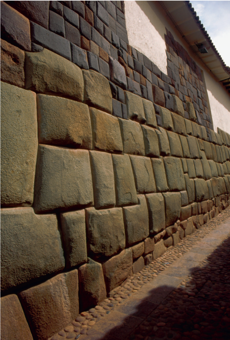
INCA STONEMWORK. In the former Inca capital, Cuzco, Peru, the Spaniards incorporated these earthquake-resistant foundations into their own buildings. © Jeremy Horner/Corbis .
