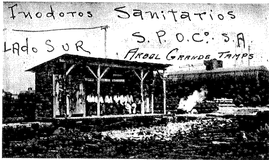
Restrooms, South Side
